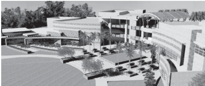
Cuyamaca College Communication Arts Building
